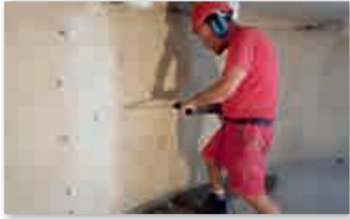
Verpressung von Rissen in Fundament- kellern Grouting of cracks in foundation cellars
