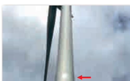
Fertiggestellte Abdichtung in Turmfarbe Completed sealing in tower colour
