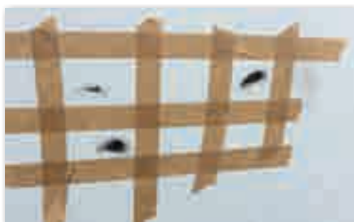
Ableben von partiellen Schadensbe- reichen Masking out partially damaged areas
